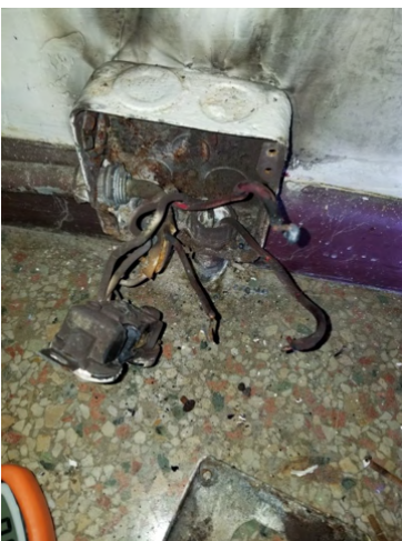
(Clockwise from upper left) Damage to wooden dance floor after dry out; Wooden dance floor boards lifting after dry out; Wooden dance floor immediately after flooding ; Wooden dance floor and hall prior to hurricanes and flooding; one of the many burnt out electrical outlets damaged by the flooding.
