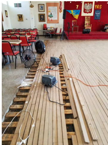
(Clockwise from upper left) Damage to wooden dance floor after dry out; Wooden dance floor boards lifting after dry out; Wooden dance floor immediately after flooding ; Wooden dance floor and hall prior to hurricanes and flooding; one of the many burnt out electrical outlets damaged by the flooding.
